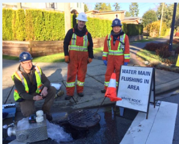
Picture 3: Water Operators performing watermain flushing.
