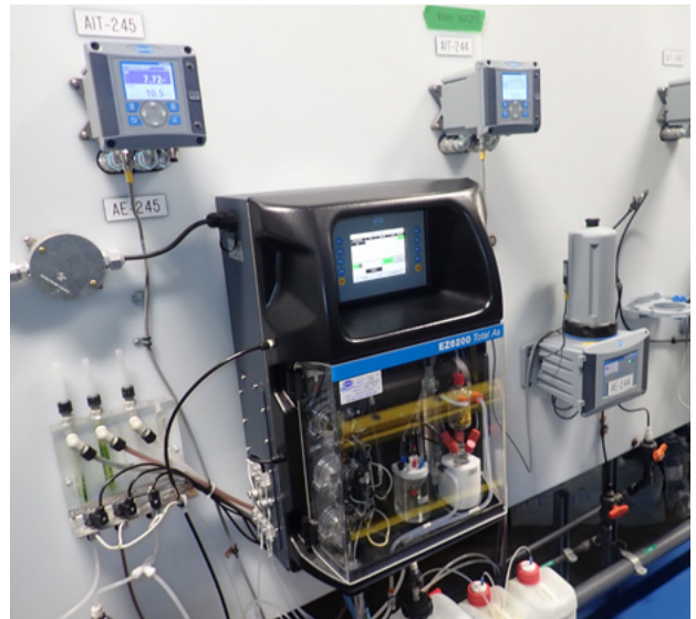
Figure 6 – Online chemical analyzer
