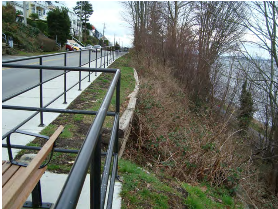
Photograph 6: Wood Crib Wall near 15191 Marine Drive
