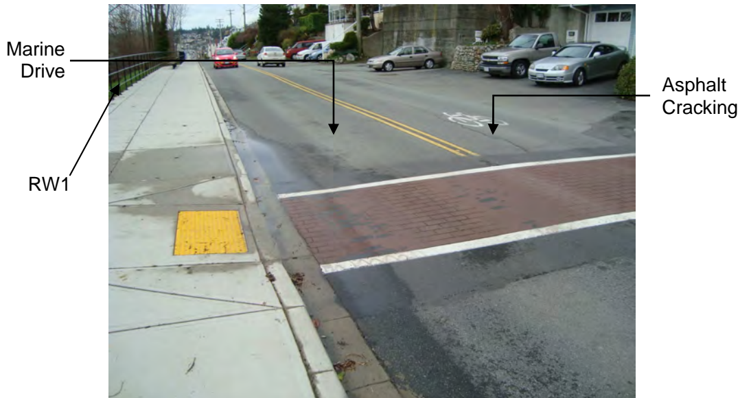
Photograph 3: Asphalt Cracking Along Marine Drive Behind RW1
