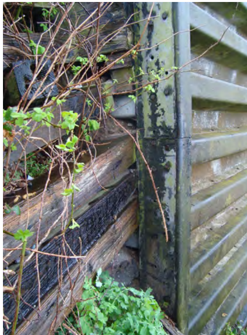
Photograph 5: Wood Crib Retaining Wall and RW1
