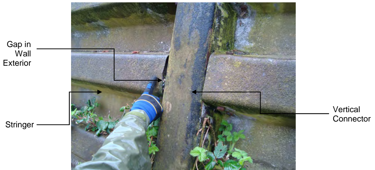
Photograph 4: Representative Gap in RW1 Exterior Facing
