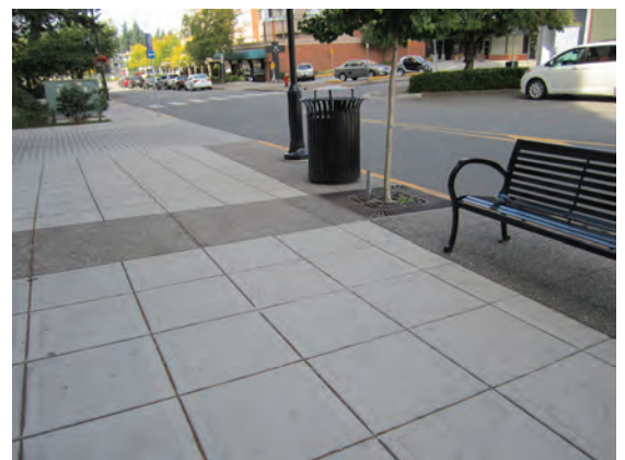
Johnston Road Paving
