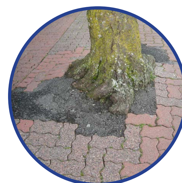
DAMAGED STREET TREES
