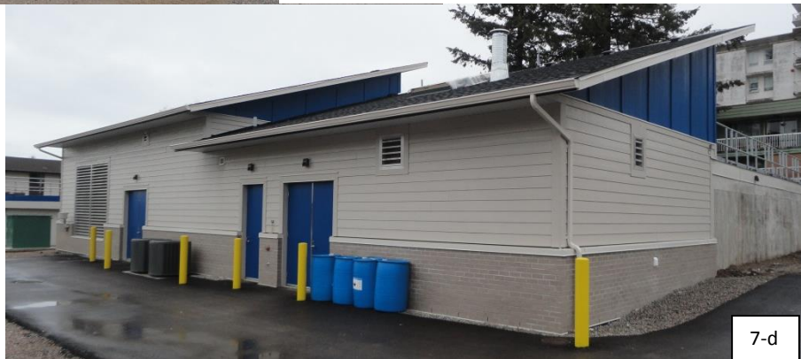
Figure 7 c&d: Merklin Reservoir close to completion
