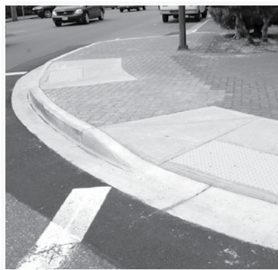
New curb letdowns on Fir
