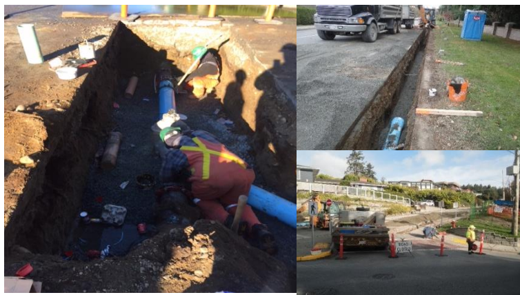
Imaae 6 - Water Main Replacement
