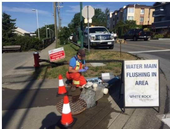
Image 8: Water Main Flushing in progress
