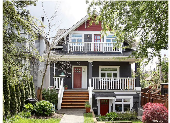
Guidelines a, b, and c: A top/bottom duplex with front veranda and balcony has a similar mass and form to a traditional single-detached home.
