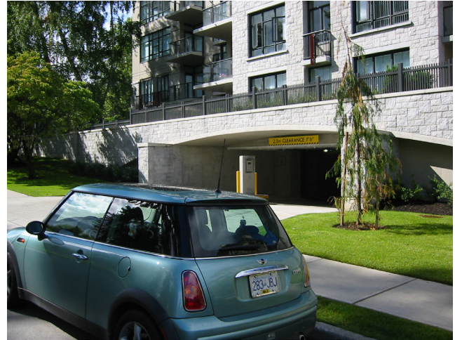
Guideline a: Parkade entrance softened by landscaping
