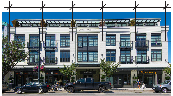
Guideline f: Facade articulation and narrow store fronts with entrances at regular intervals
