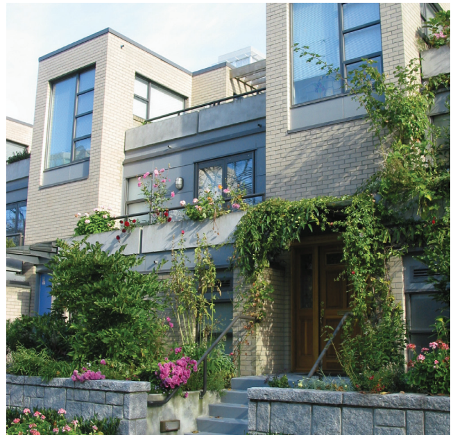
Guidelines c and j Massing and natural materials are varied to break up the building front and create visual interest
