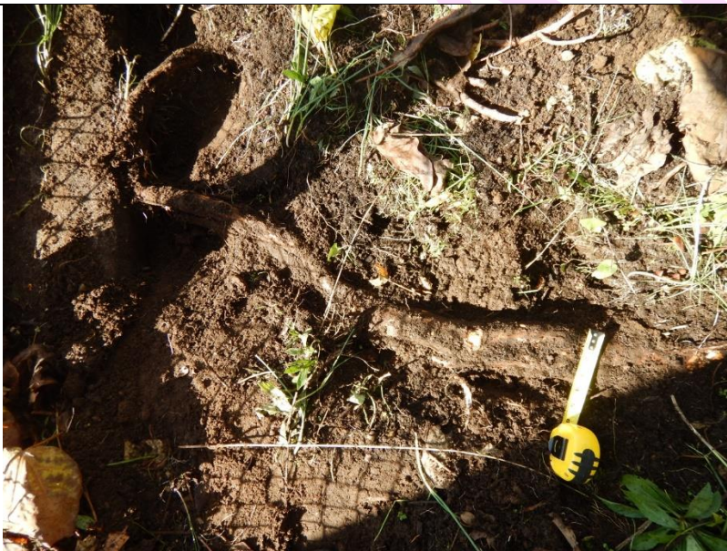
Figure 4. Intact roots on the south side of the tree, measured 1.0 m north of the retaining wall.
