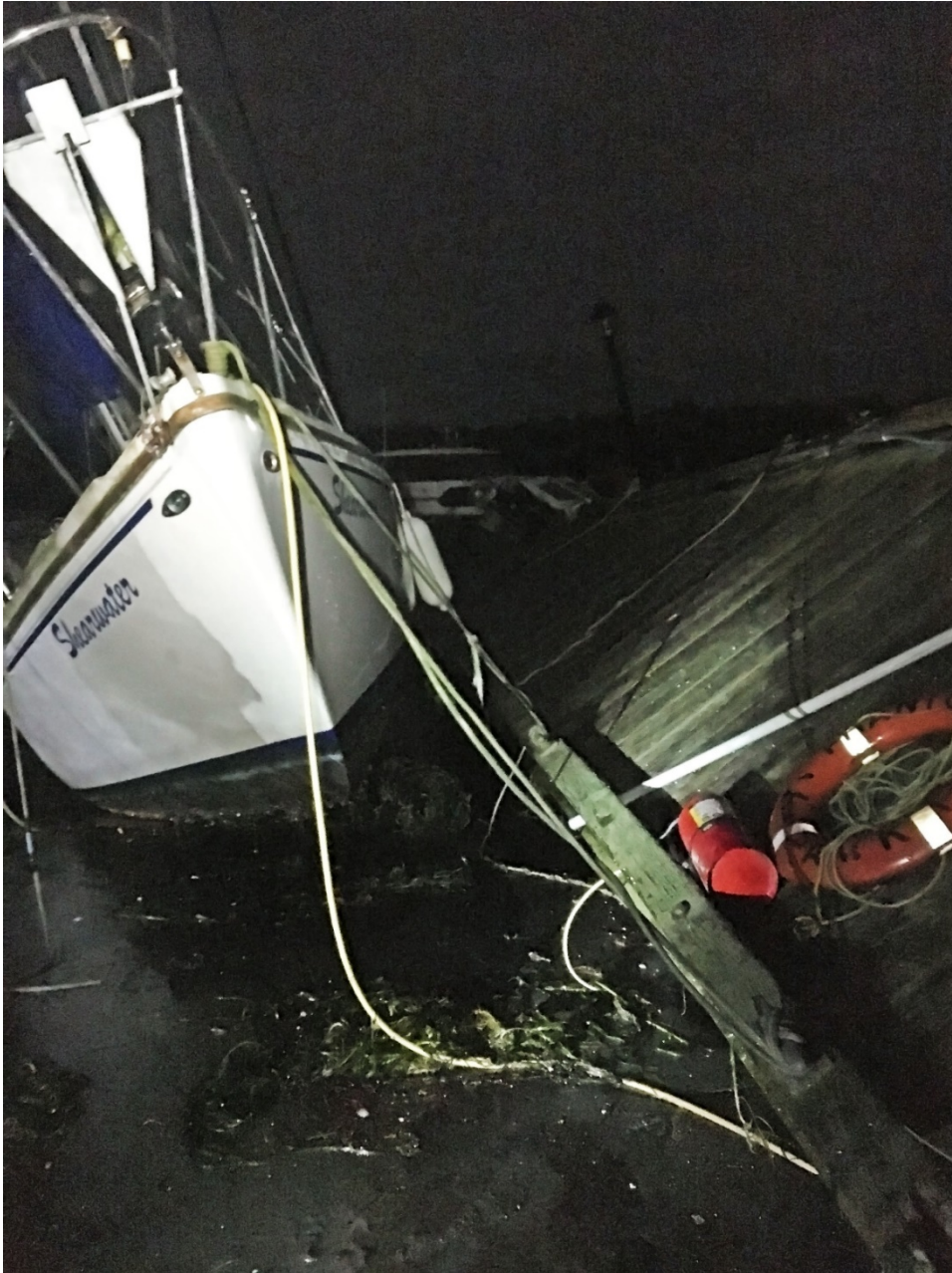
Photo 5: Failed section of West Marina Float
