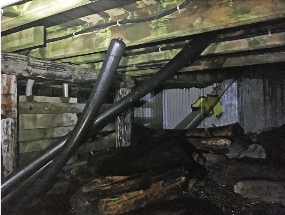
Photo 8: New services installed near shore abutment
