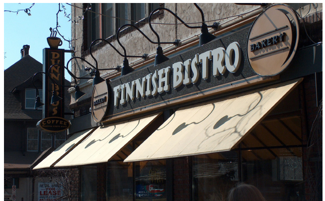
Guideline i: Duckbill lighting is used to highlight signs and building entrances in retail areas
