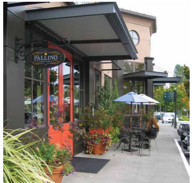
Guidelines c, d, g and k: Windows and colour variations along the front elevation, weather protection above the entrance level with the sidewalk, and projecting signage
