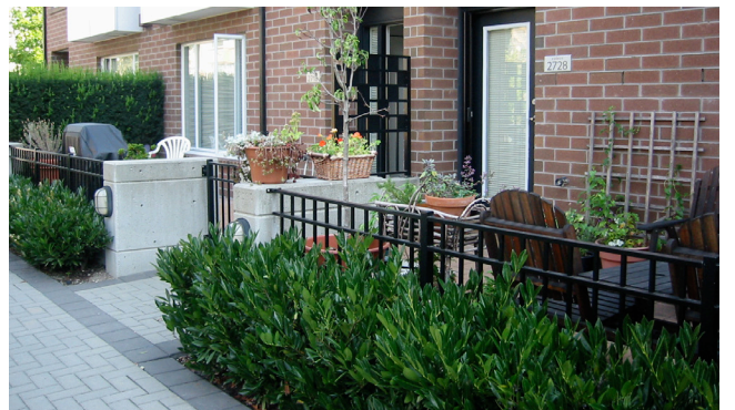
Guidelines b, g, and i: Ground-oriented units, entrances directly off of and level with the sidewalk, natural materials, and private outdoor space
