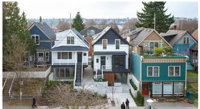
Guideline a, b, and c: Up/down duplexes, with parking at the rear and share pedestrian access to reduce paved area, reflect the established streetscape by incorporating pitched roofs, front porches, and similar materials and fenestration
