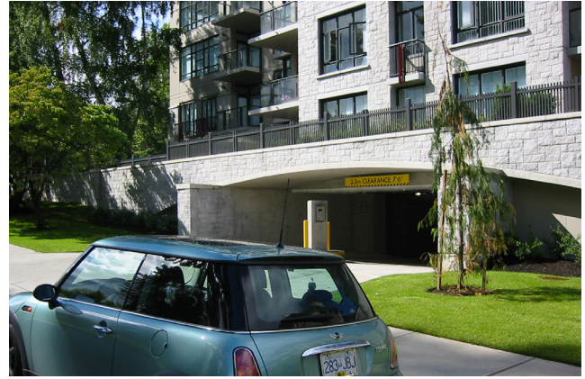
Guideline a: Parking entrances are designed to be discrete and softened by landscape.
