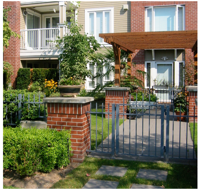
Guideline d: Main entrances are level with the sidewalk, and residential units on the ground floor are ground-oriented.
