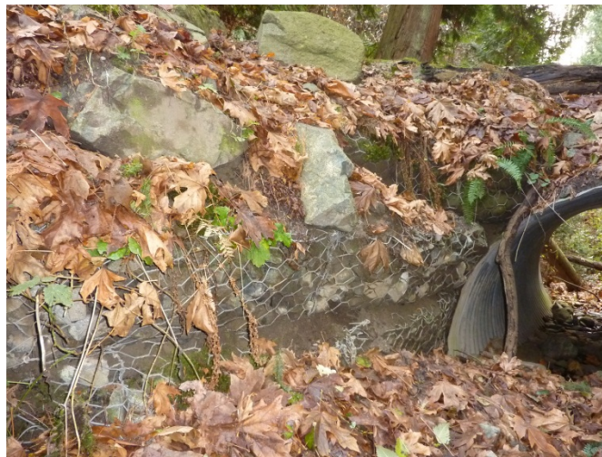
Photo 6 Duprez Ravine – Gabion Wing Wall at Culvert Footbridge Inlet
