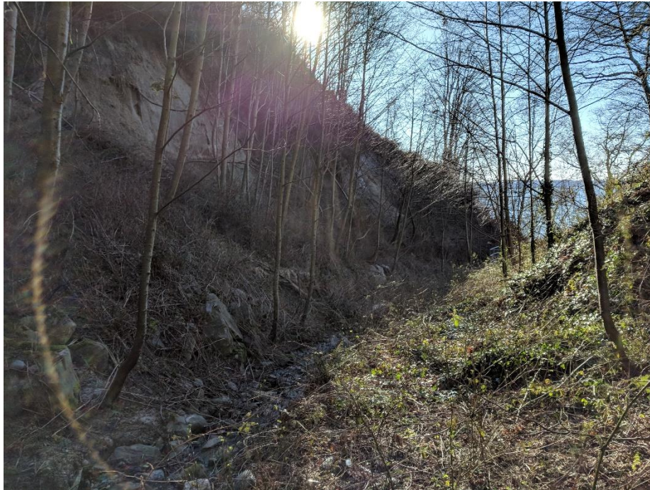
Photo 1 Lower Coldicott Ravine - Near-vertical Soil Face on East Ravine Slope
