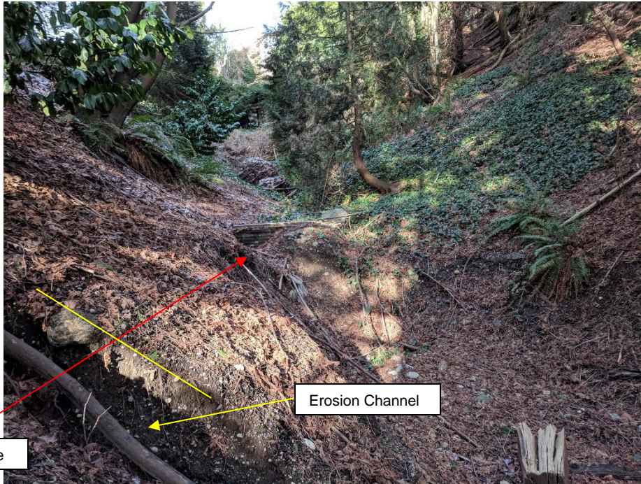
Photo 15 Everall Ravine West Branch – Erosion at bottom of Ravine
