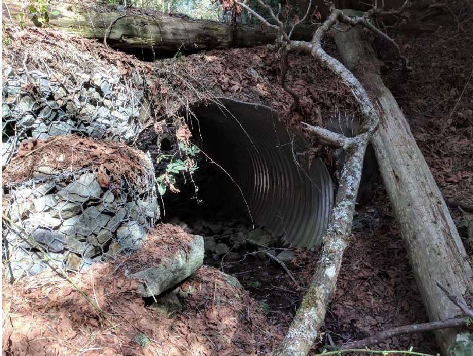
Photo 11 Duprez Ravine – Gabion Wing Wall at Culvert Footbridge Inlet
