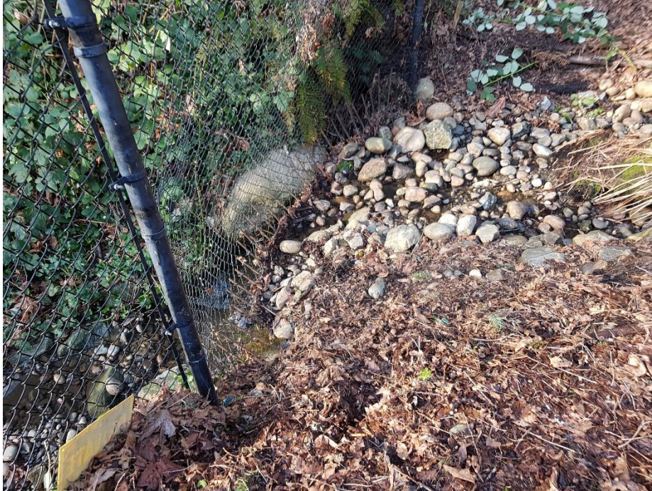
Photo 19 Everall Ravine – Rebar Reinforcement for Fence
