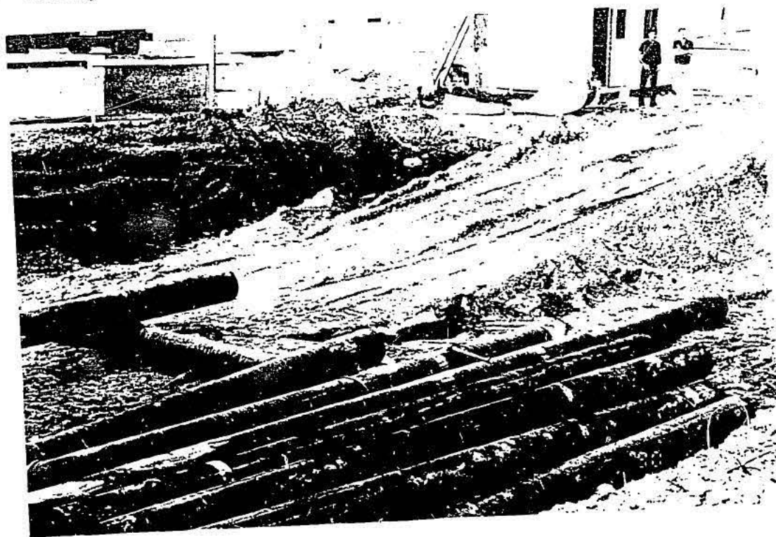
2. Looking towards the southwest. Excavation walls show some organics mixed with the native silt material. Aug. 25, 1990.
