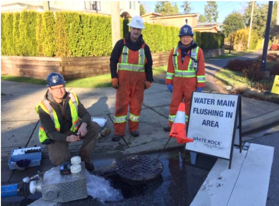
Figure-6, The Water Department Operators conducting the Unidirectional Flushing program
