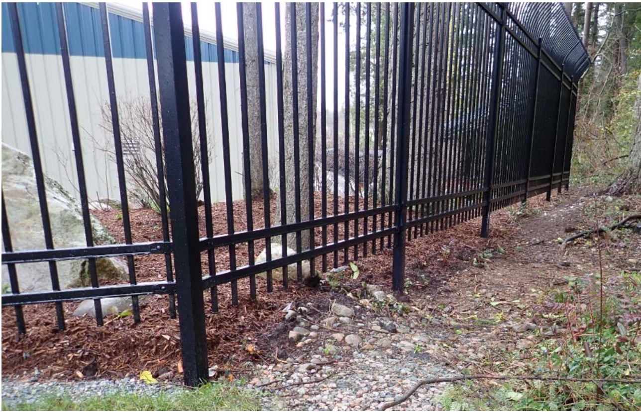
Figure-3, Fence Construction for the White Rock Water Treatment Plant
