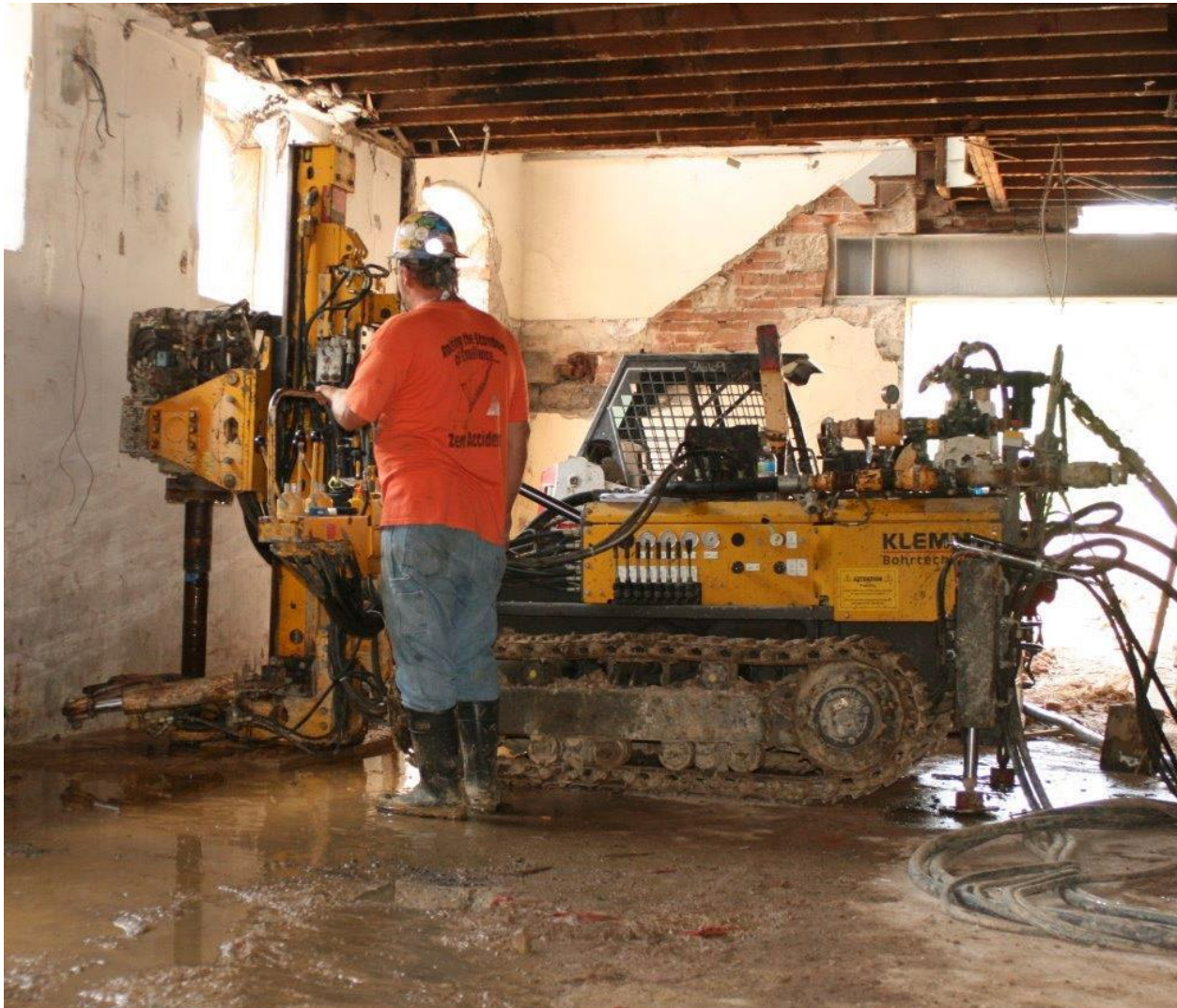
Figure 1 – Equipment for installation of micropiles ( https://www.haywardbaker.com/uploads/solutions-techniques/micropiles/ )
