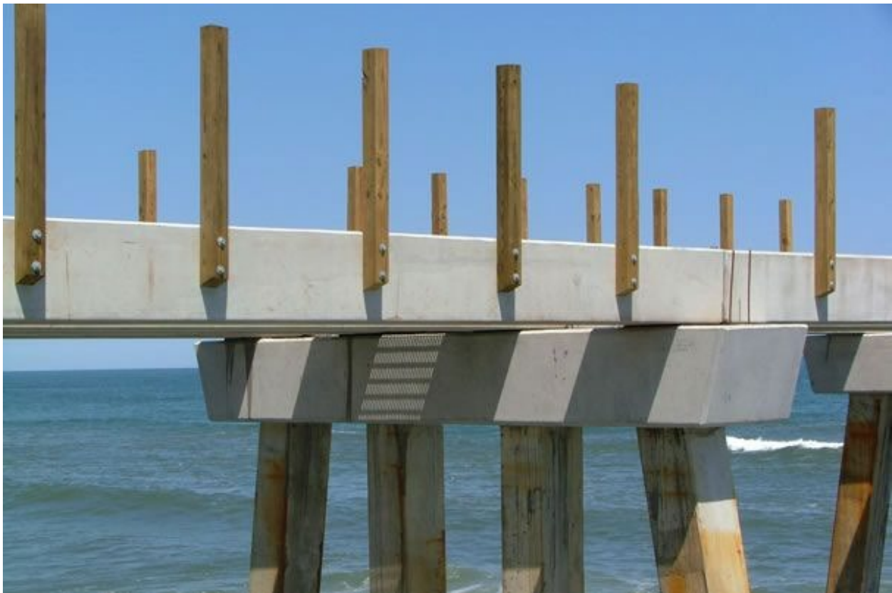
Figure 3 - Concrete Pile and Deck Structural System
