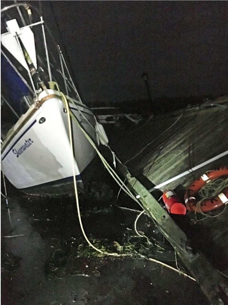
Photo 5: Failed section of West Marina Float
