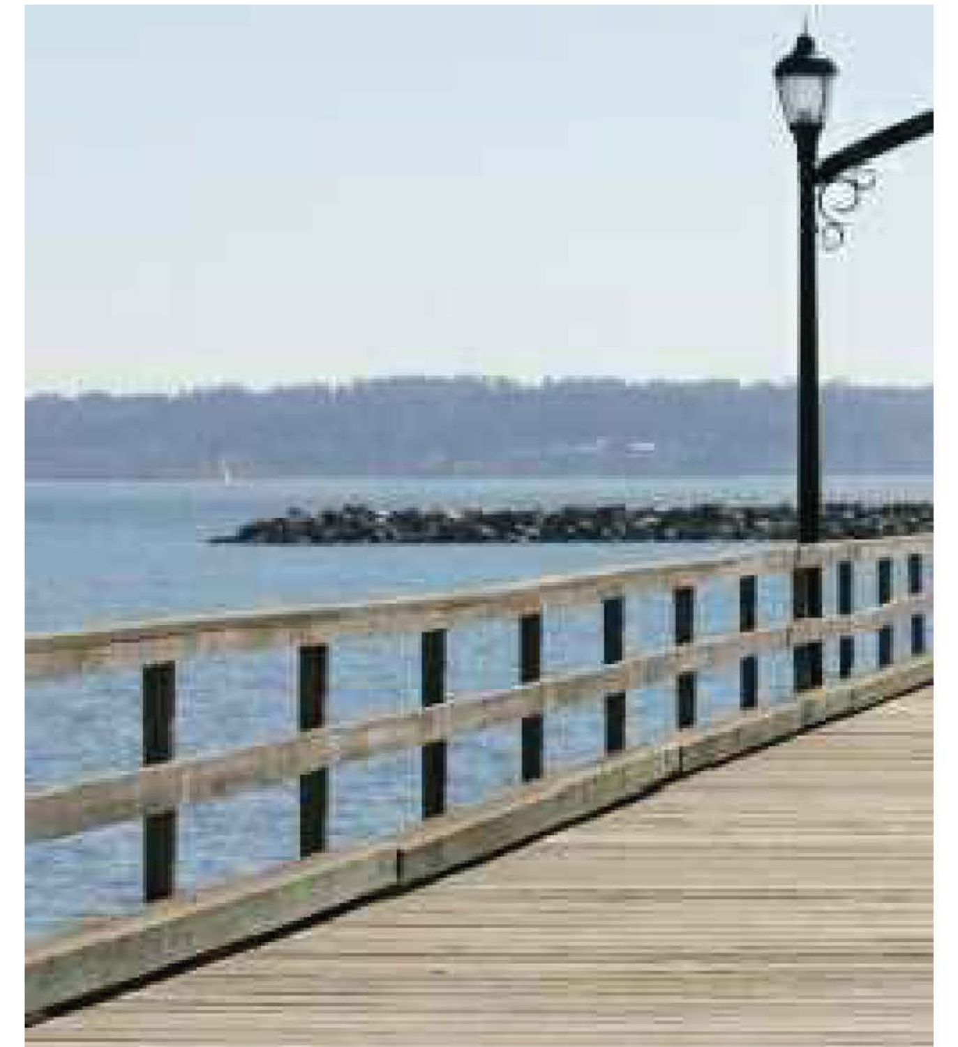
EXISTING PIER HANDRAIL
