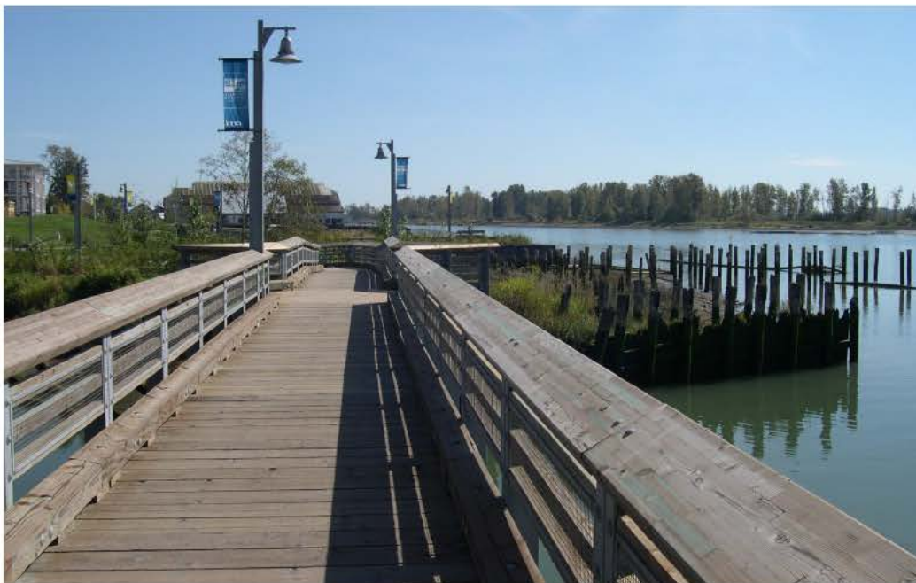
Figure 9 – Example of proposed code compliant handrails.
