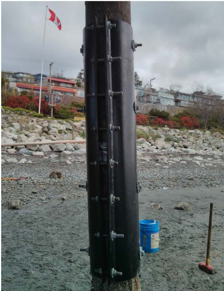
Figure 8 – Installation of Jackets around piles
