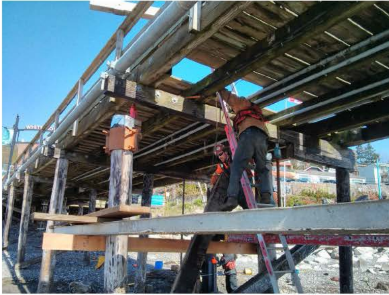
Figure 4 – Temporary shoring of pile bents
