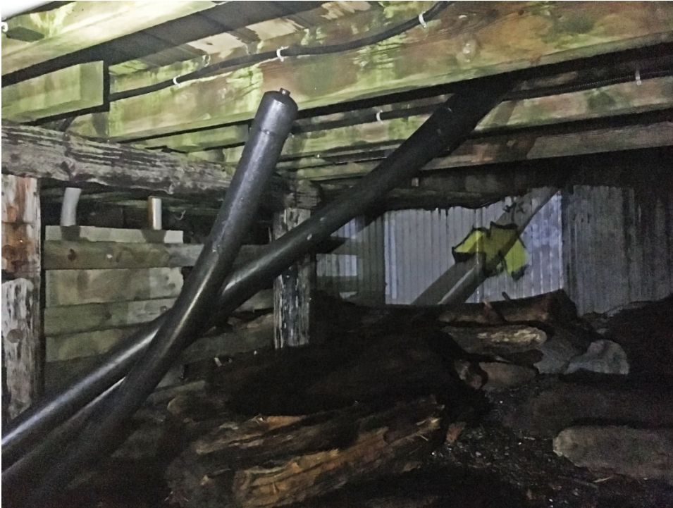
Photo 8: New services installed near shore abutment
