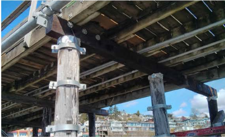
Figure 7 – Steel Clamps around Piles
