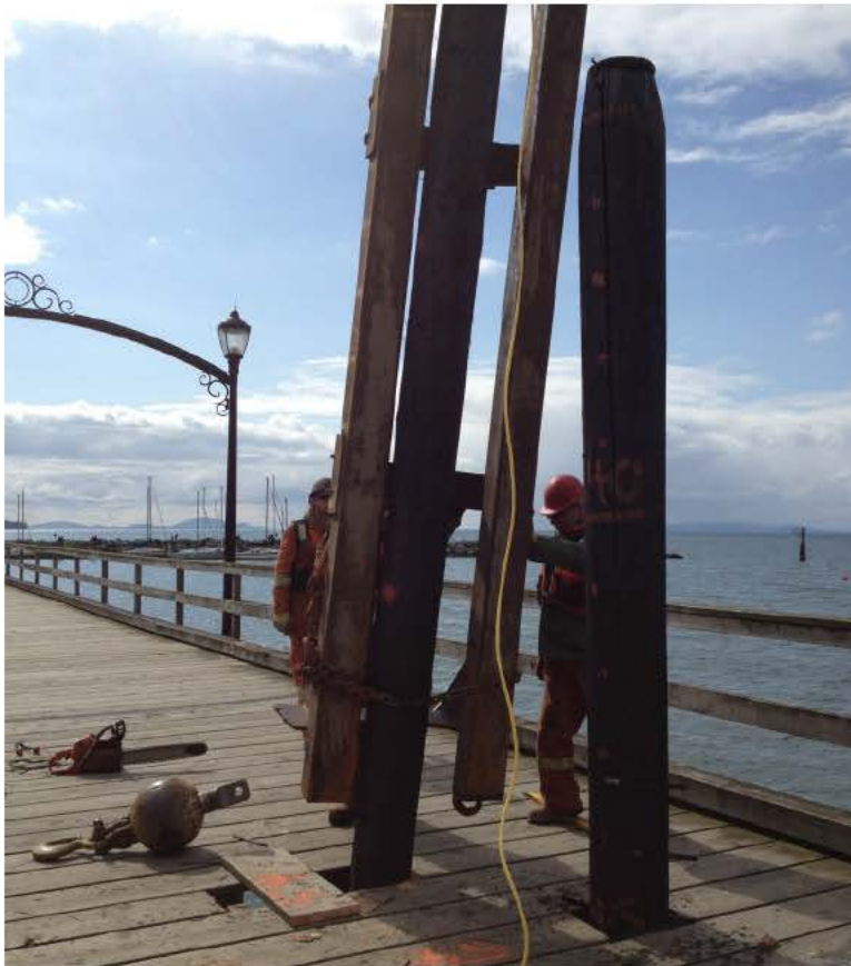
Figure 5 – Localized removal of deck to install piles
