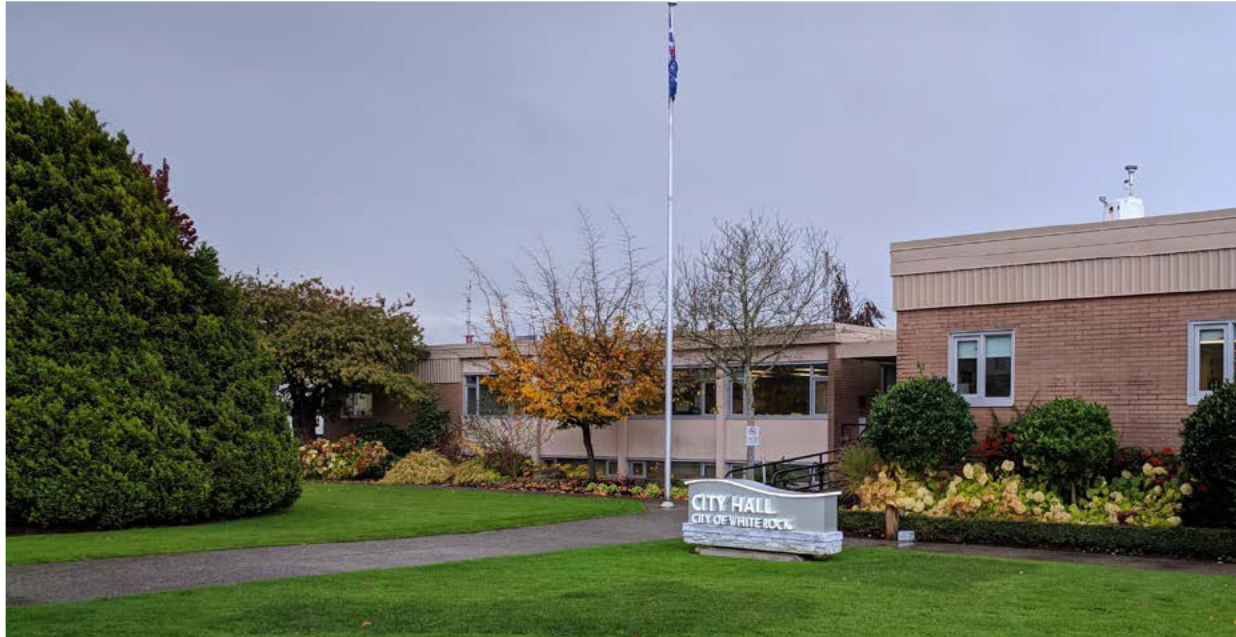
Figure 1: North Elevation of White Rock City Hall
