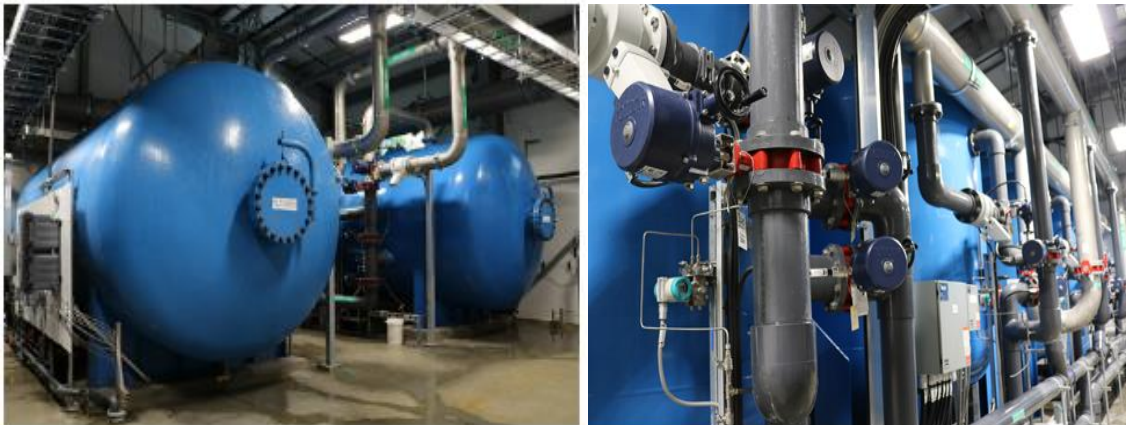
Figure-11, The newly constructed White Rock Water Treatment Plant
