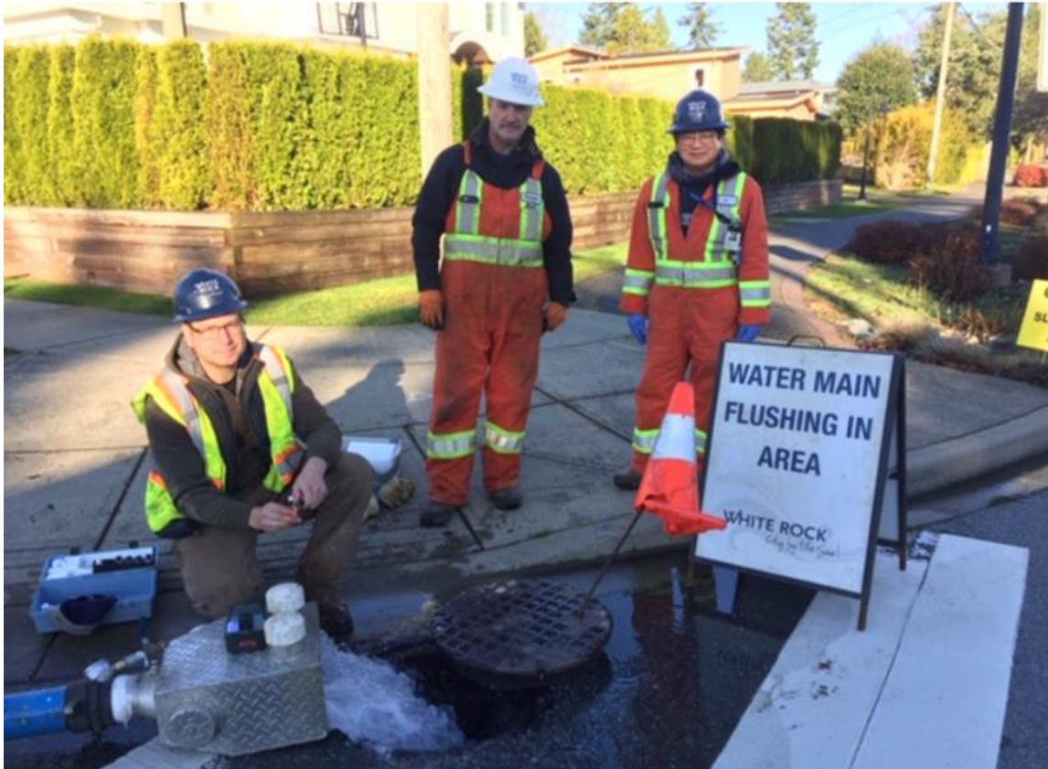
Figure-7, The Water Division Operators conducting the Unidirectional Flushing program
