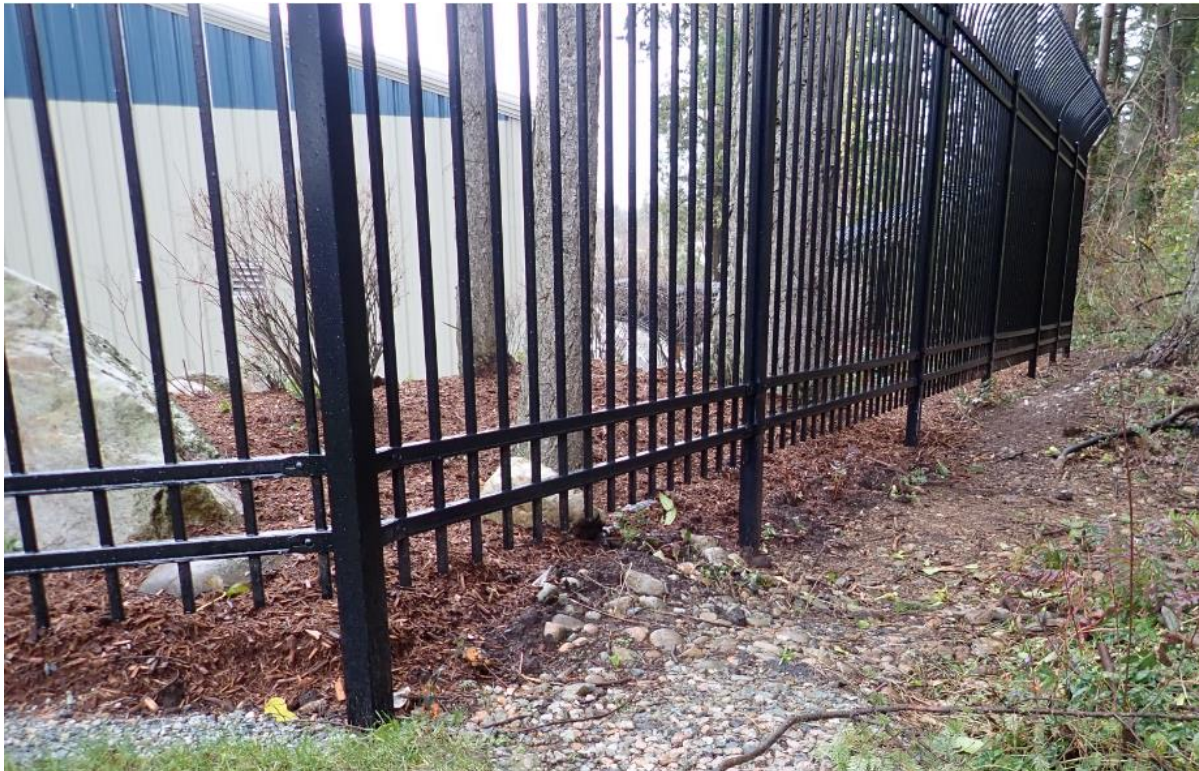
Figure-5, Fence Construction for the White Rock Oxford Water Facility
