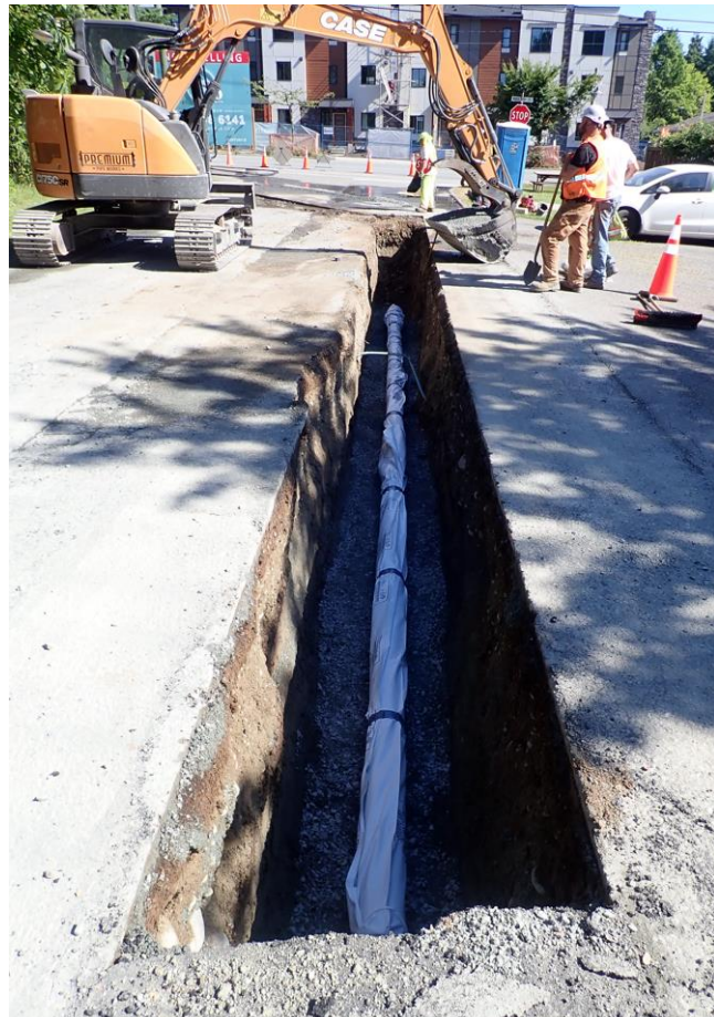
Figure-10, Stevens Street watermain construction
