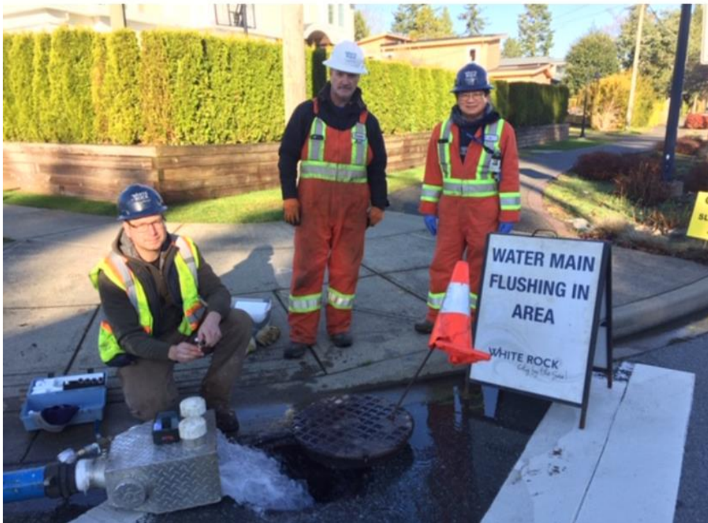
Figure-6, The Water Division Operators conducting the Unidirectional Flushing program
