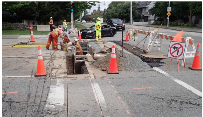
Figure-12, North Bluff Road/Best Street Intersection. Connection of White Rocks Water Utility to Surrey's Water Utility.
