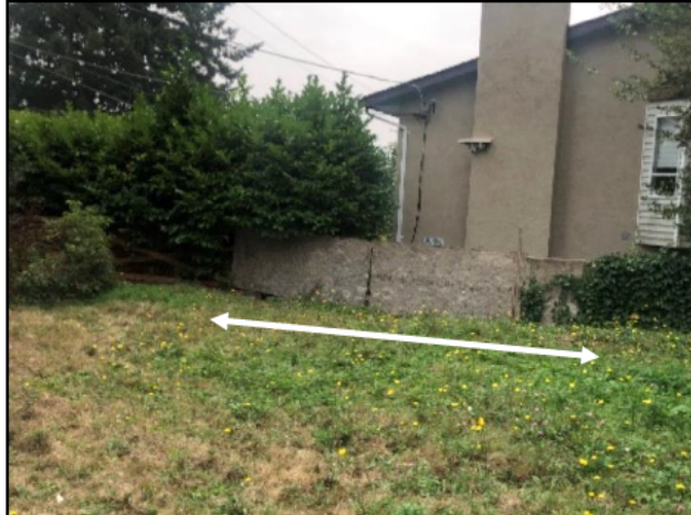
Fig. 15 – North property line of 1441 Vidal St, east corner.
