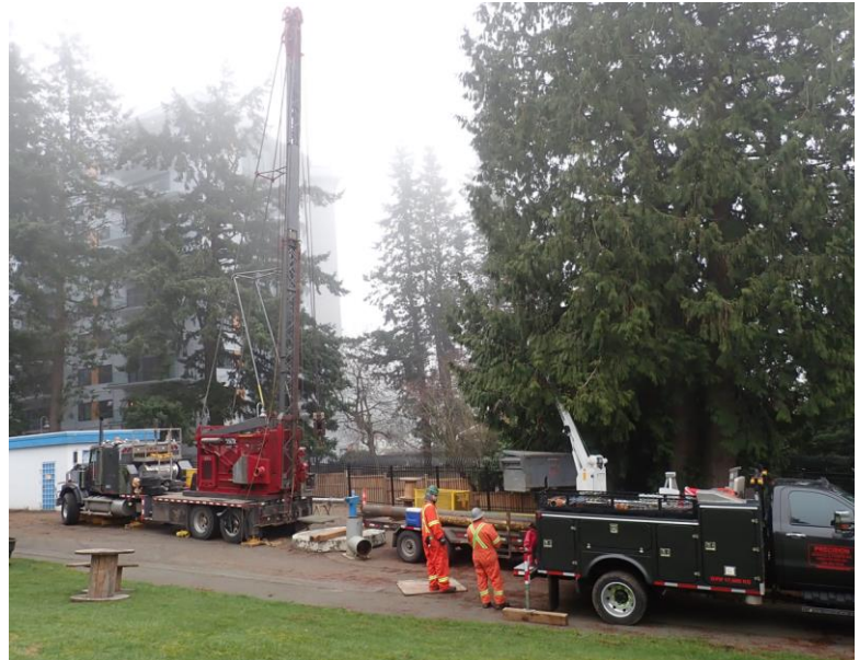
Figure 11 - Redevelopment at Well #1, Oxford well field.
