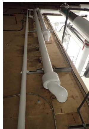
Figure 13 - Completed Pipe insulation above plant offices
