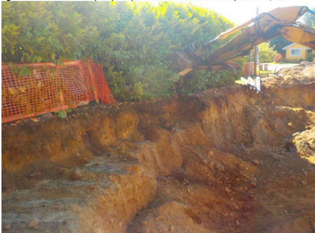
Figure 5. Excavation of foundation around OS1 September 26, 2017
