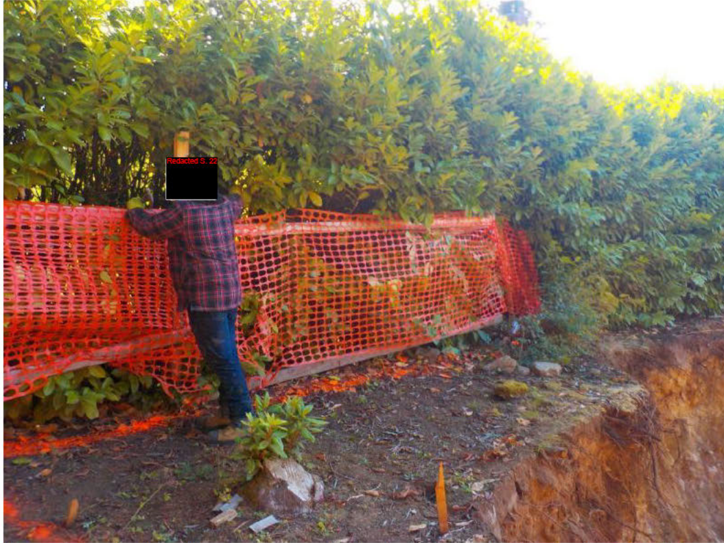
Figure 4. Construction of temporary tree protection barrier around OS1 September 26, 2017
