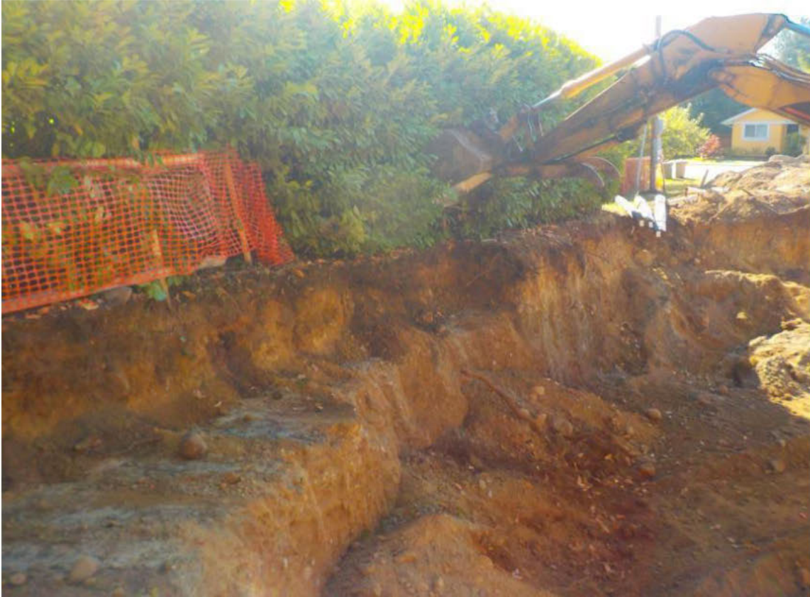
Figure 1. Excavation of foundation around OS1 - September 26, 2017
