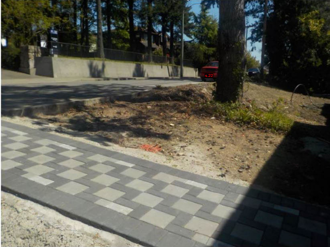
Figure 11. Completed walkway – May 8 2020.
