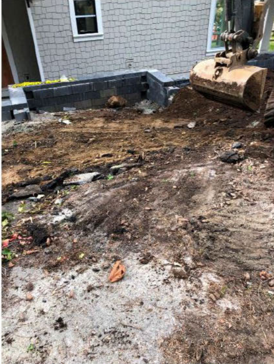
Figure 4. Removing asphalt – April 2, 2020.
