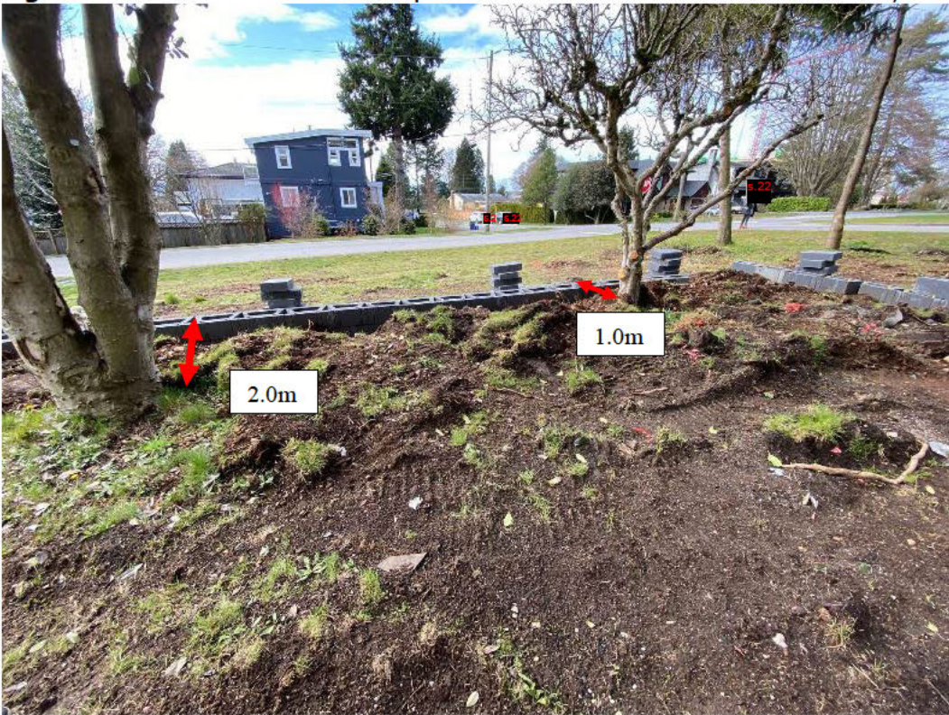
Figure 22. Tree 2408 & 2409 – Retaining wall installed south side at 2.0 and 1.0m respectively – March 16, 2022.
