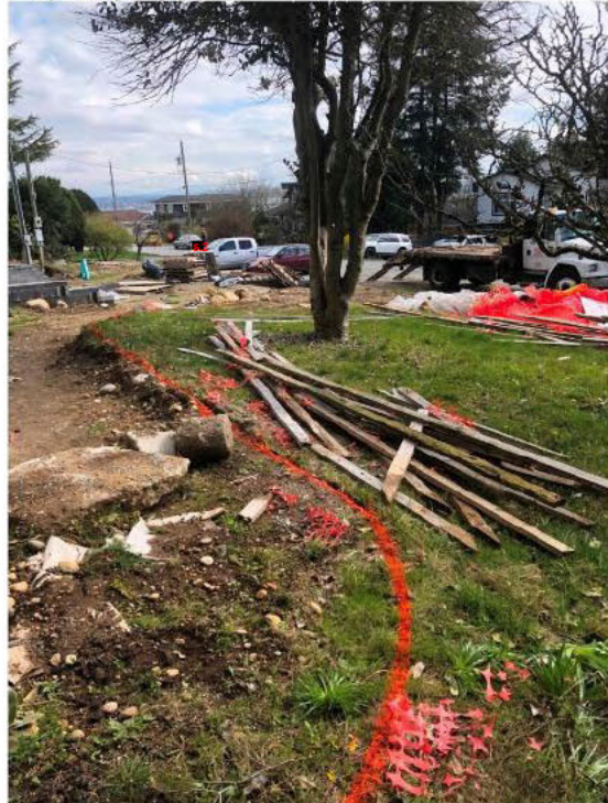
Figure 10. TPZ's spray painted to mark machine 'no-go' zones – April 2, 2020.
