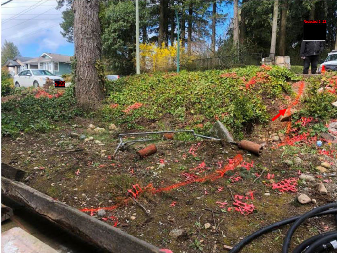
Figure 6. Old concrete stairs removed – April 2, 2020.
